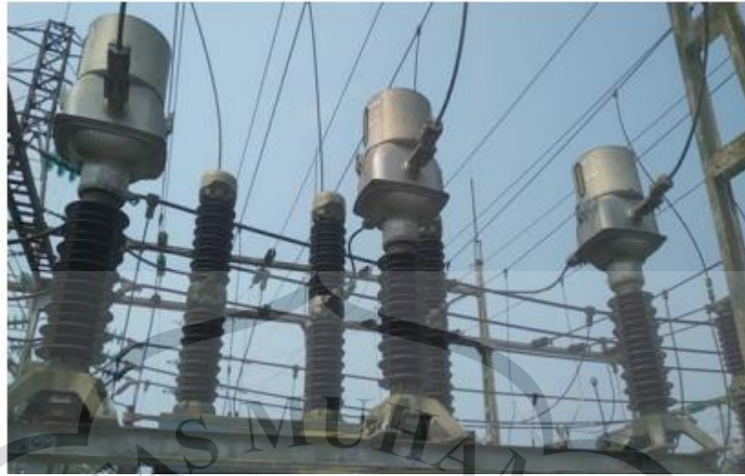
Gambar 2.2 Current Transformer (CT) (Tolibin, 2025).
