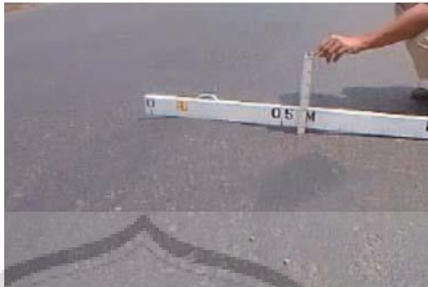
Gambar 2.2 Alur (Rutting)
