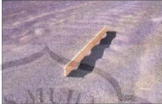
Gambar 2.1. Keriting ( Corrugation ) Sumber : Bina marga no.03/MN/B/1983
