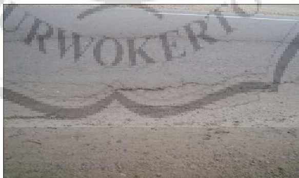
Gambar 2.5 Cekungan ( Bumb and Sags ) Sumber : Bina marga no.03/MN/B/1983
