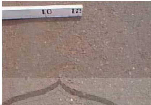
Gambar 2.13 Pengausan Agregat ( Polised Agregat ) Sumber : Bina marga no.03/MN/B/1983
