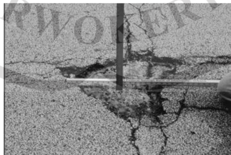
Gambar 2.17 Lubang
