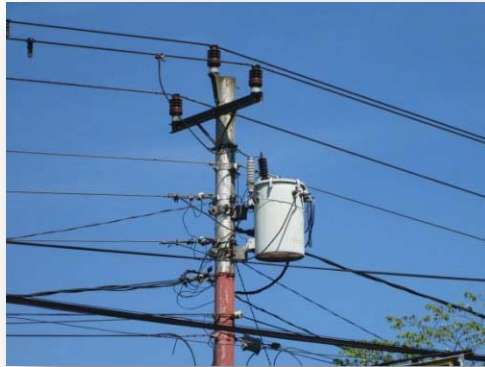
Gambar 2.2 Transformator distribusi 1 phasa
