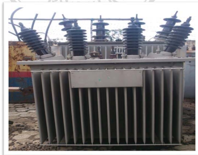
Gambar 2.3 Transformator distribusi 3 phasa
